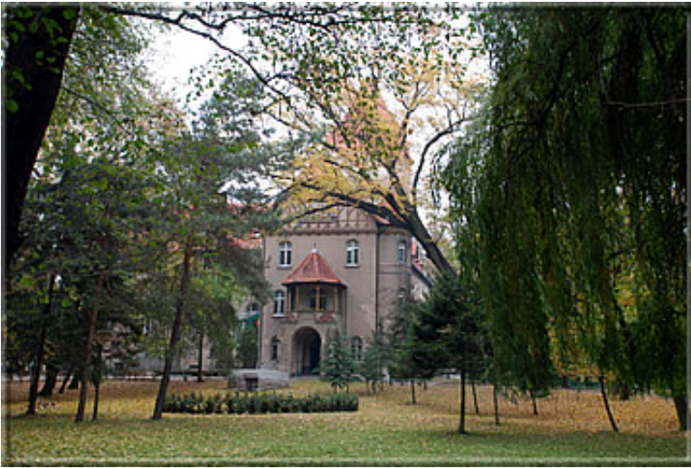
... and a further partial view (west wing)
