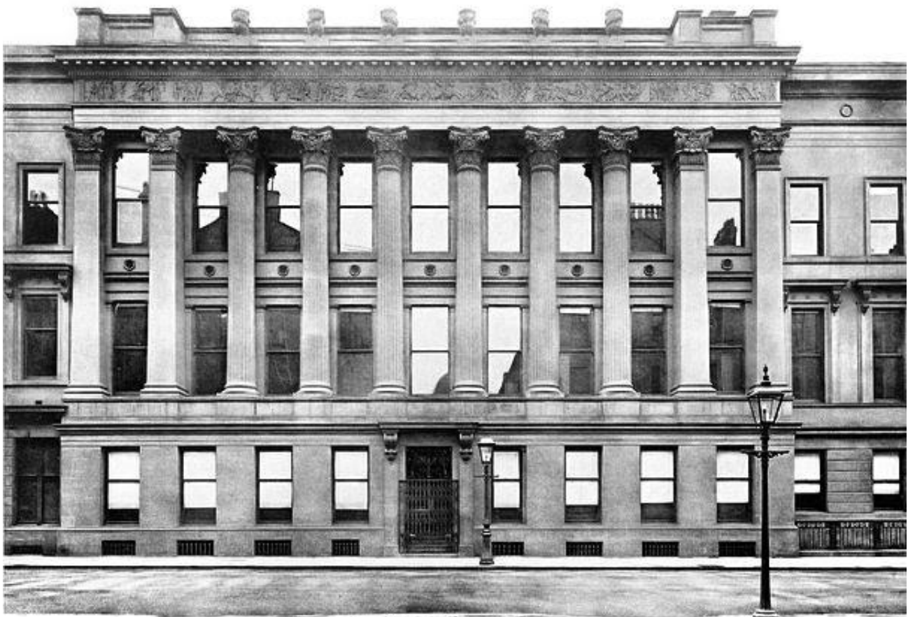
THE MUNICIPAL AND COUNTY BUILDINGS, GLASGOW. MESSRS. CLARKE AND BELL, ARCHITECTS, 1844.
